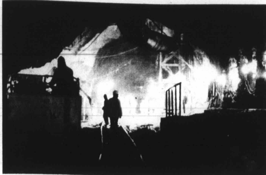
DEEP TUNNEL WORK — Work goes on in the 200-foot deep Metropolitan Sanitary District's Deep Tunnel project under Chicago and surrounding communities. A citizen's group has asked for halt on the project, which is being constructed to control pollution and flooding. Cost of the project has risen from original estimate of $1.6 billion to $7.3 billion.
