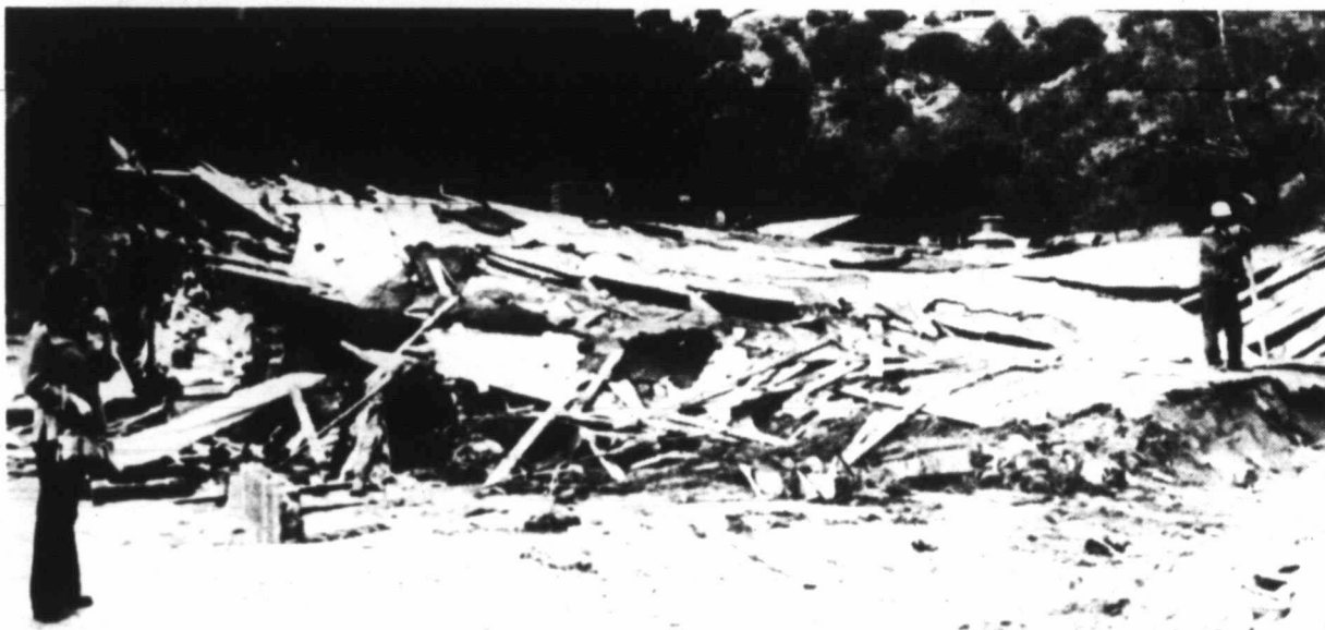
RUINS — Townsfolk survey ruins of Hidden Springs lodge, Hidden Springs, Calif. Sunday where officials are still searching for bodies of missing victims from Friday's flood. Shortly before the water hit Friday many residents were fighting a fire at the lodge. Several met their deaths and some barely escaped.
