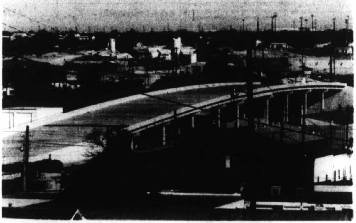
NEW APPROACH — This is the new overpass connecting Highway 350 and also traffic from IS 20 with the old Highway 80 at 3rd Street. It was long awaited in Big Spring and completed this
