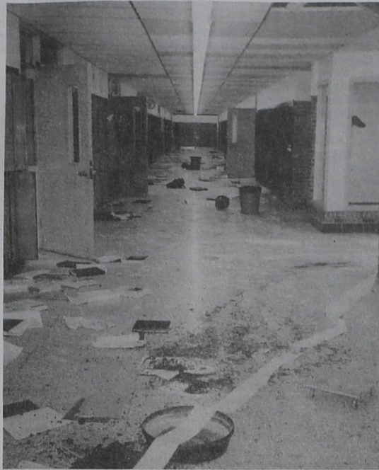
SCHOOL RAN-SACKED.... One of the hallways at Friona High School is shown as school and law officials discovered it early Thursday morning. Vandalism really "did a number" at the school. Friona ISD is offering a $500 reward for the arrest and conviction of the responsible parties.
