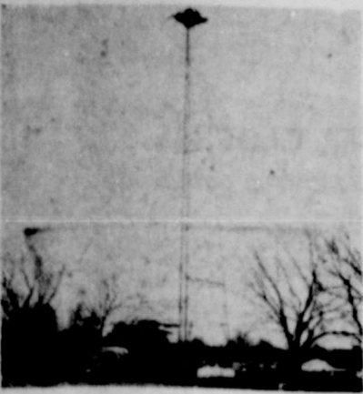
136-FOOT DERRICK at American Liberty's No. 1 D. A. Fellers "tight" test well a mile north of the city limits.
