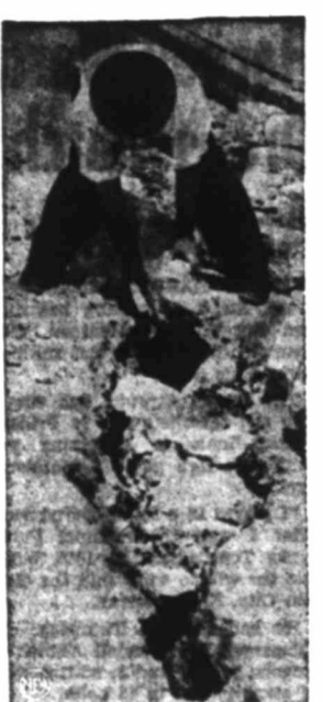
CRACKED EARTH — A village on the Greek island of Zakynthos uses rocks, shattered masonry and any other available debris to fill the earth cracked by earthquakes. The quakes, which imposed the arduous task of rebuilding ruined communities, took more than a thousand lives throughout the Greek Ionian islands.
