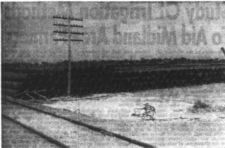
STANTON STOREHOUSE — Some 25 miles of 30-inch pipe has been unloaded at Stanton for use in the Permian Basin Pipeline Company Spraberry gas outlet project. In the top picture, some of the valuable pipe is stacked awaiting pick up by trucks (bottom picture) for the trip to the field where it will be strung along the 96-mile Midland to Denver City right-of-way.
