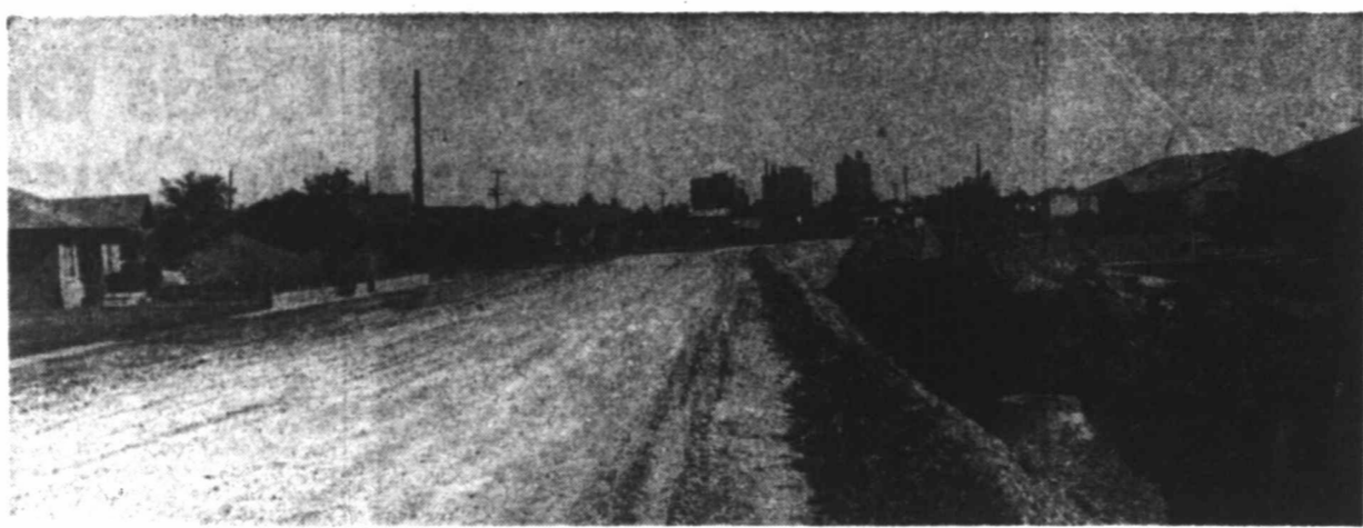
North Big Spring Street lies agape as storm sewer is laid.
