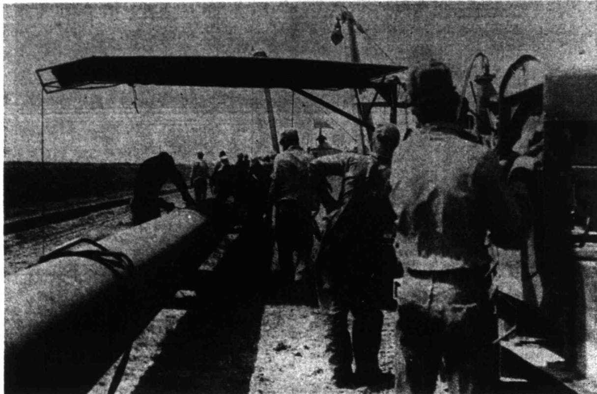
PIPE KEEPS MOVING —Welders, shielded from the blistering sun, kept up their fast pace Tuesday as foot after foot of pipe began stretching through the Spraberry Trend Area. A Periman Basin Pipeline Company project, the network of pipe and plants will re-
