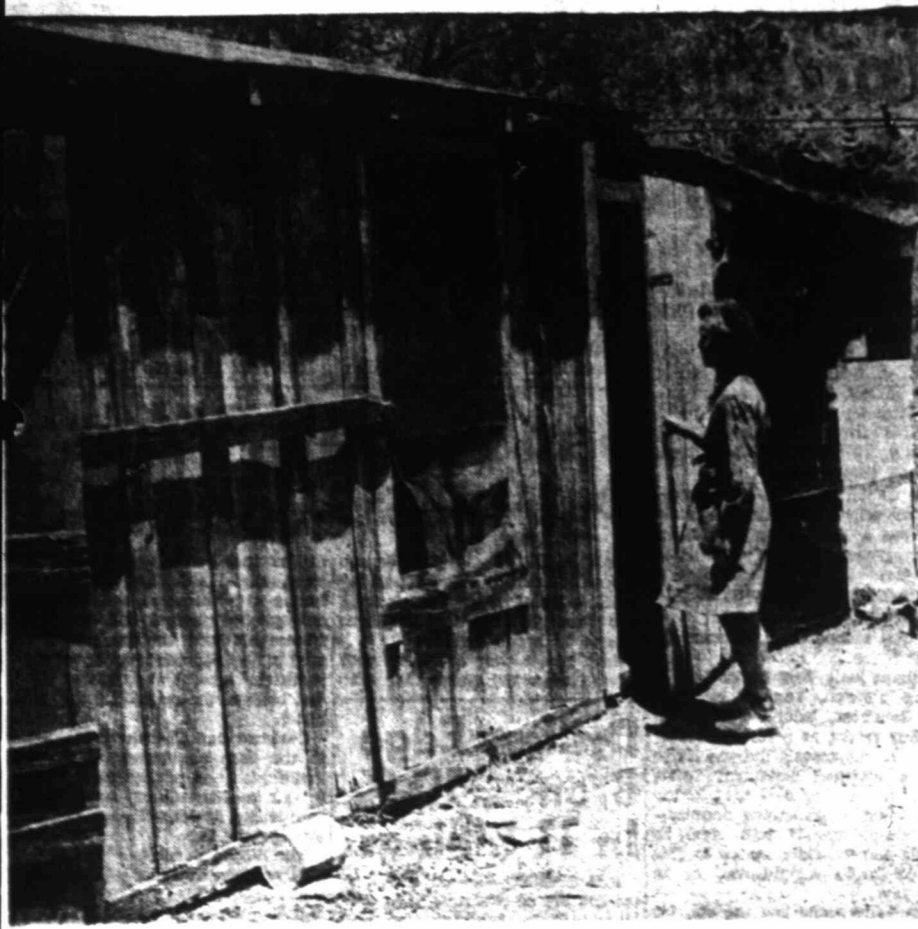
GIRL SCOUT CAMP BUILDING —A Brownie Scout prepares to enter one of the shelters at the Mitre Peak Girl Scout Camp in the Davis Mountains. The Permian Basin Council has started its building fund campaign in an effort to raise $125,000 for repairs and improvements to the campsite, which is presently inadequate to provide facilities for all the girls in the 15-county area.
