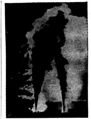
STEAM FROM NATURE'S BOILER—Here, resembling small oil gushers, are two steam bores in Wairakei, New Zealand Scientists are boring 1500 feet below the earth's surface in an attempt to harness underground steam which they hope to use to
