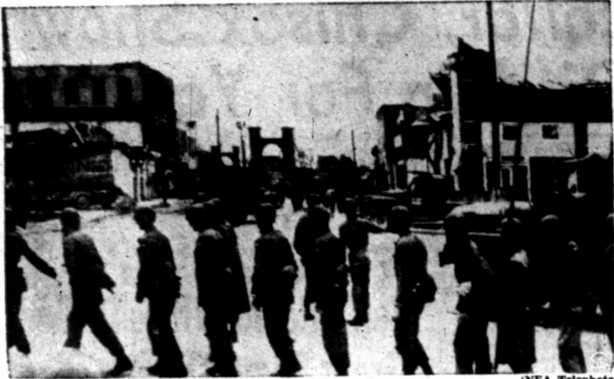
CLEAN-UP ENGAGEMENT —Troops of the First Armored Division stationed at Fort Hood arrive in Waco to engage in clean-up operations in the tornado-stricken city. Gateway to Waco's old suspension bridge, condemned after the tornado, can be seen in the background.
