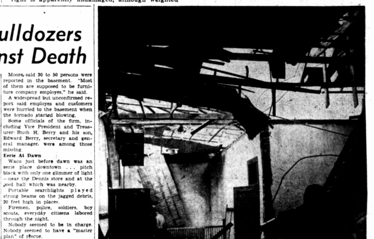
SCHOOL ROOM'S DESTRUCTION—Hazy sunlight filters through the gaping hole of one of the rooms of the Lake View School, after Monday's tornado made off with its roof. Much of the roof toppled to the interior of the section. Almost 1,000 youngsters at the school miraculously escaped death in the storm thanks to the discipline of the teachers and youngsters themselves who laid down on the floor in the hallways.
