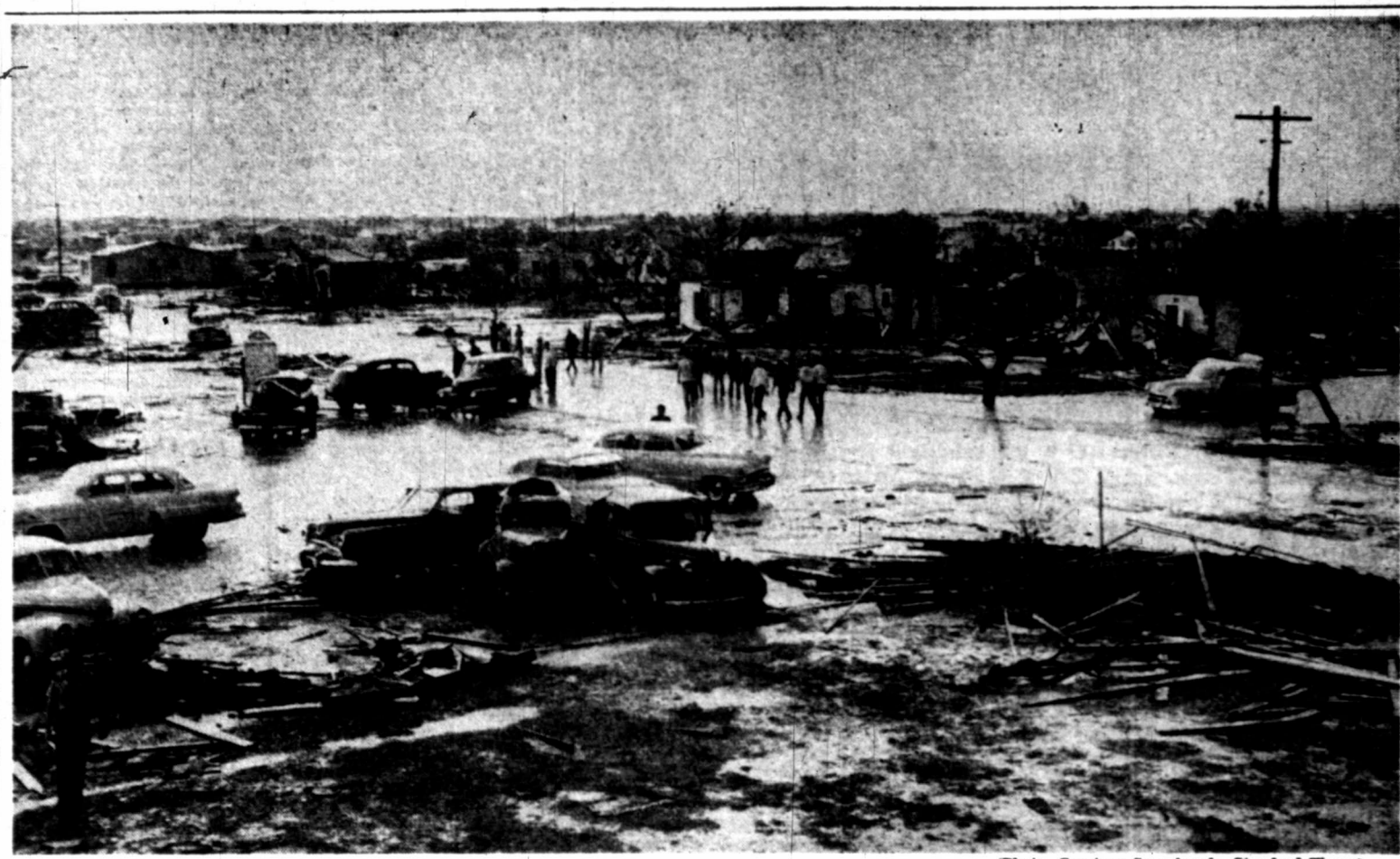
AFTER THE STORM —A view from the direction of the Lake View High School in San Angelo shows the destructive force of the tornado which caused hundreds of thousands of dollars in damage as evidenced by the shells and remnants of scores of residential buildings lying in the half-mile-wide, two-mile-long, east-west swath of the twister. These torn and twisted automobiles, surrounded by splintered timber and shredded metal roofing are mute evidence of the devastation. Rapid water flow and mud hampered vehicle passage for disaster teams and debris generally added other potential danger to the general area. Fast falling rains plus an electric power shutoff helped prevent further spread of the disaster by fire. (Photo Courtesy San Angelo Standard-Times.)
