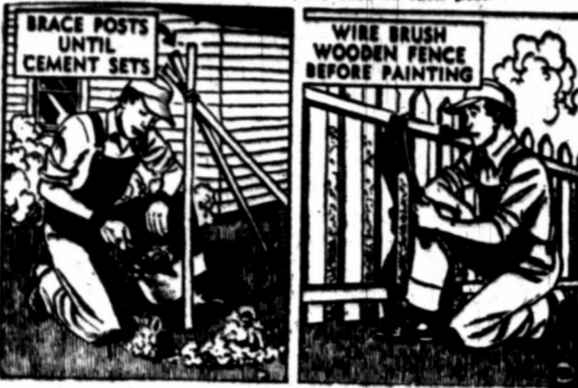
To prevent deterioration of wood or metal fences, keep a good coating of paint on them, set fence posts in concrete.
