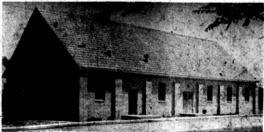
First Christian Church's new Youth Building.
