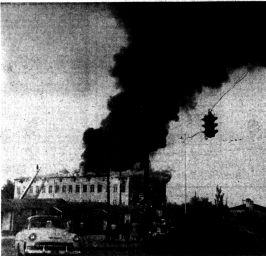
CHURCH BUILDING LOST IN FIRE —Black smoke rises from the Educational Building of the First Baptist Church Sunday as Midland firemen carry water hose to the top of the structure. Flames broke out on the third floor, and two hours later had caused damage estimated at $150,000. It was Midland's biggest fire in more than a year.
