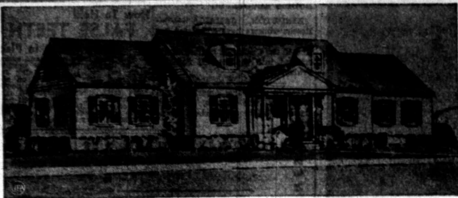
'MAMIE'S CABIN' —During presidential golfing vacations at the Augusta National Country Club in Georgia, President and Mrs. Eisenhower will live in a $40,000 six-room brick cottage, shown in architect's sketch. The retreat, informally dubbed "Mamie's Cabin," is being financed by the club.
