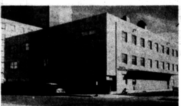
SHEP DID THE ROOFING —The Shepard Roofing Company offers the solution to your roofing problems. The fine workmanship of the firm solved three major problems in its roof job on the new Midland National Bank Building.
