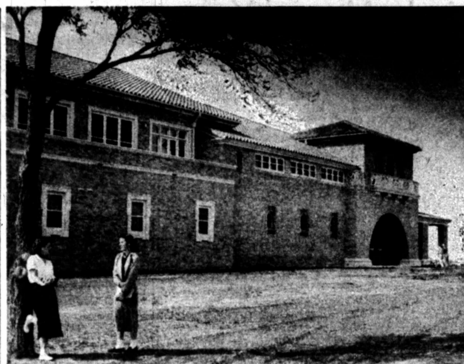
NEW TEXAS TECH STUDENT UNION —This half million dollar Student Union Building, latest addition on the Texas Tech campus, will be opened formally April 12. Though students have been using the building since March 10, the public will get its first look at the building at the open house. Two years in the building, the Student Union sticks to the Spanish Renaissance architecture of the campus, but the interior is of comfortable, modern design.
