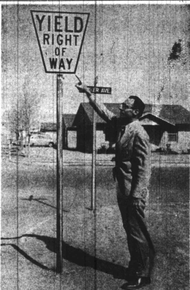
'YIELD' SIGNS INSTALLED —City Traffic Engineer Jack Keese points to one of the new-type "Yield Right-of-Way" signs installed for tests at six intersections here. Motorists approaching on Marienfeld Street have to stop at Parker Street only when there is approaching traffic. If the roadway is clear, they may proceed without stopping. Observations will determine whether the signs will be used throughout the city.
