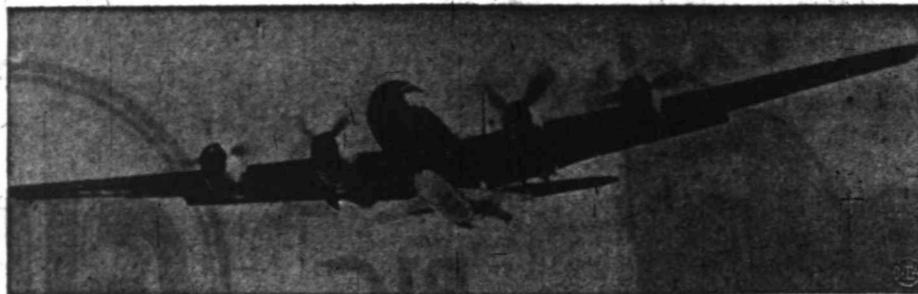
AERIAL HITCHHIKER —With "baby" fastened securely in place, a specially modified B-29 takes to the air at Seattle, Wash., prepared to launch the tiny Douglas Skyrocket at a high altitude. Once dropped from the mother ship, the pilot of the small plane ignites his rockets, and in an hour's time, the small ship has attained a speed of 1233 miles per hour and altitude of 75,494 feet.
