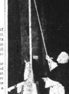
**HEAT BEACON**—The unique heating device, above, is being used in the Church of Santa Maria Delle Grazie, in Milan. Many of Italy's old churches were built before the development of central heating, and are uncomfortable on cold winter days. The "heat beacon" houses a container of bottled gas, and plates at the top of the device beam heat to all parts of the church as the plates revolve.
