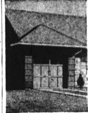
This garage is under the same roof as the house, but a hip roof-style projection over the garage adds variety to the design. Asphalt shingles are blended.
