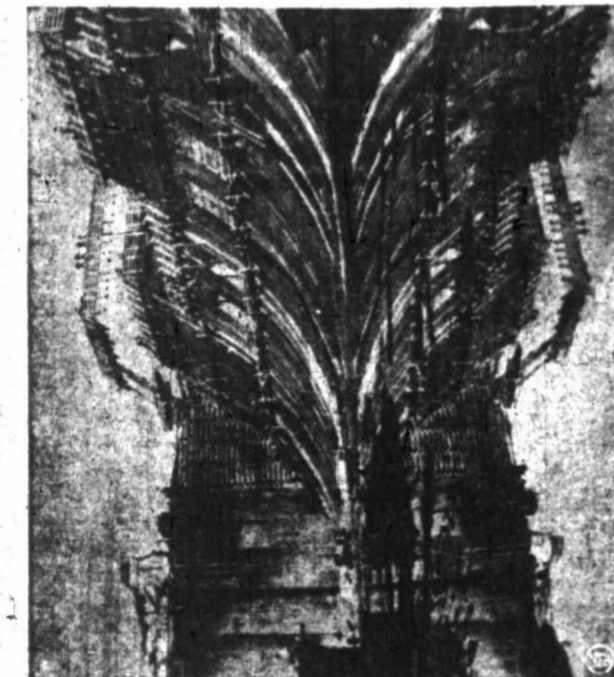
BIG DAM ILLUSION —This may look like the prow of a ship under construction, but it's just an illusion. Turn this page one-quarter turn to the right, and you'll see Chief Joseph Dam, at Bridgeport, Wash., mirrored in water covering the concrete "floor" of the downstream spillway. When completed, the dam will play an important part in the flood control of the Columbia River.
