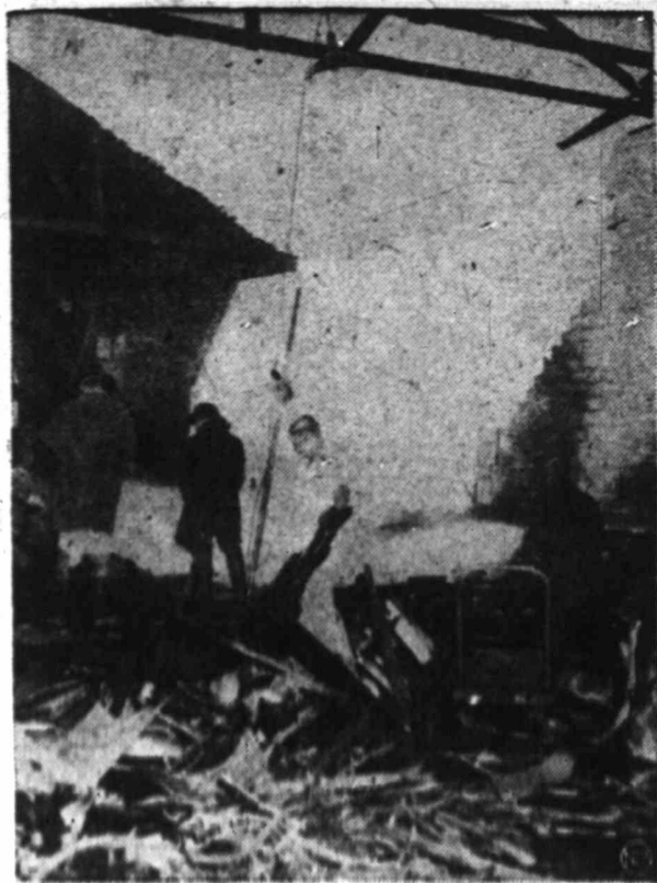
(NBA Telephone) EXPLOSION RIPS PLANT — Volunteer firemen search debris in a Bell Aircraft Plant warehouse just north of Fort Worth following a fire and explosion that wrecked the building and destroyed critical and hard-to-get magnesium castings. Ten persons were injured, none seriously. Damage to the building and Korea-bound helicopter parts was estimated at $1,000,000.
