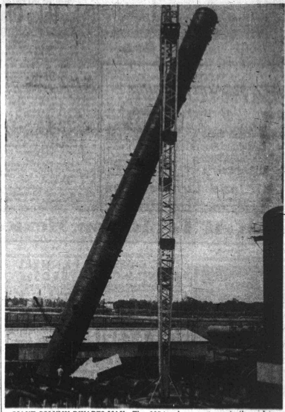
GIANT COLUMN DWARFS MAN —The 185-ton benzene concentration column which is erected at Shell Oil's Deer Park refinery dwarfs the man shown at the base of the column. The unit, 155 feet long, 9 1/2 feet in diameter was constructed in Dallas by the Foster Wheeler Corporation and transported by rail on three flat cars. The column is part of the aromatic section of the platforming unit, and required two and one-half hours to erect.
