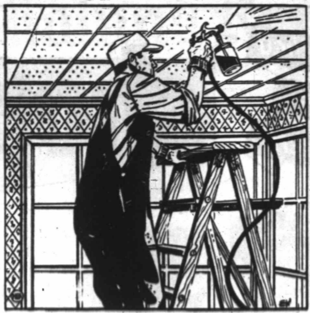
Wise homeowner, using a spray gun to paint an acoustic tile ceiling, applies a dark color to absorb light streaming in windows.
