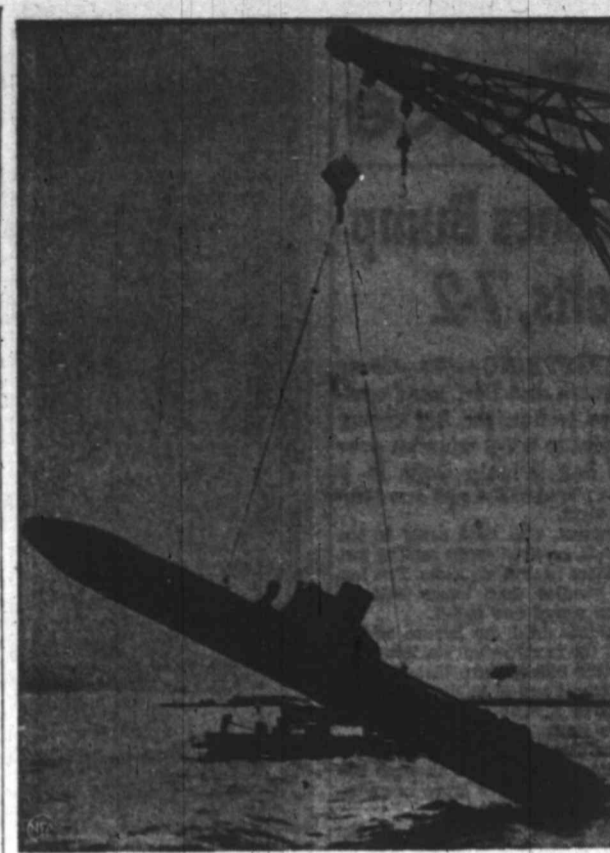
SALVAGING A SEA DRAGON —Yanked from the sea bottom after seven years, the Japanese suicide submarine, Kaityu (Sea Dragon), dangles from a salvage ship's crane off Yokohama, Japan. Suicide subs, 60 feet long, carried two-man crews and a six-foot nose full of explosive powder. Center was a 25-foot storage battery space and filling seven feet of the stern was the craft's engine.
