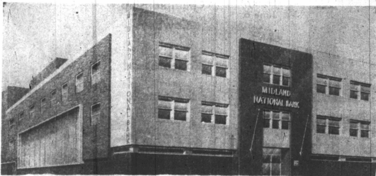
The New Midland National Bank Building Now Under Construction
