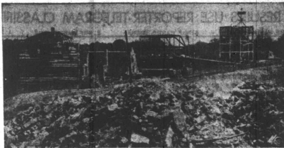
CALCULATED DESTRUCTION—More than four months of time, $200,000 in money, and the efforts of a 60-man crew have been necessary to effect this scene of wartime destruction at Olney, Md. Designed to serve as a training ground for Civil Defense workers, it embodies most demolition problems that might be met after an air raid.
