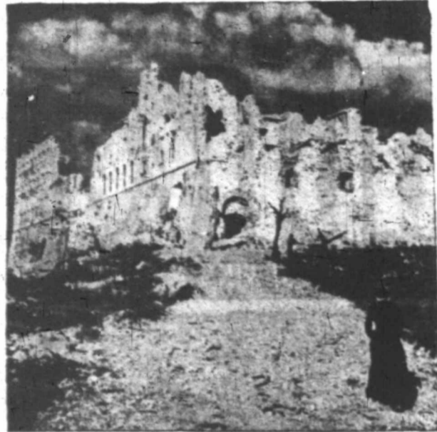
A year later, a lone priest makes his way up the rubble-strewn path. Note arched doorway in center and northern wall at extreme left.
