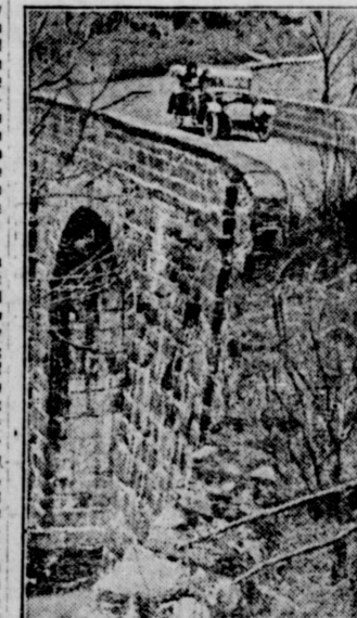
Substantial Stone Culvert.
