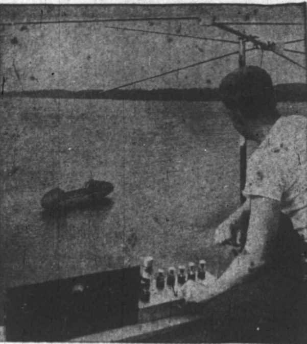
Apparently drifting without a pilot, the new lifeboat is actually responding to "orders" from the radio transmitter in foreground.
