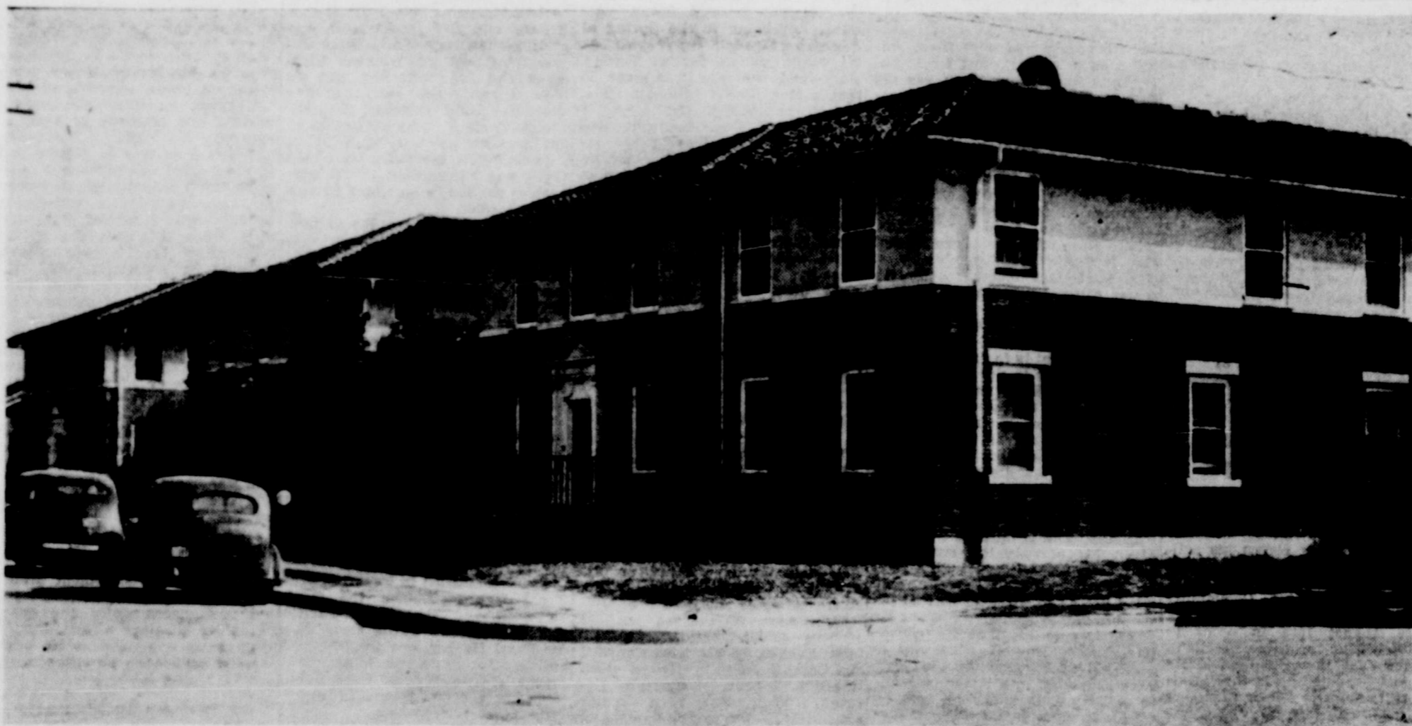
COMPLETED BUILDING TODAY, Finished at a Cost of Approximately $100,000, and Increasing Capacity to Sixty-Five Beds for Patients.
