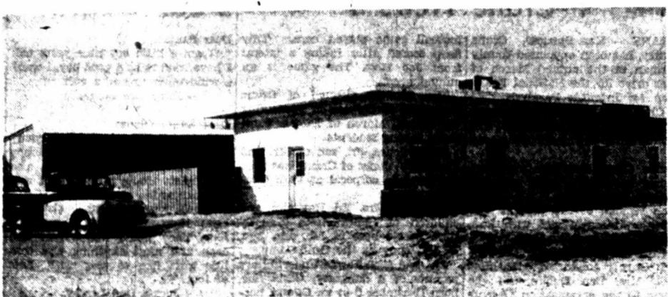
ONE-STOP SERVICE —The Mid-West Lumber Company is one-stop headquarters for all building needs. The firm also does general contracting, commercial and residential, and will repair and rebuild. Joe B. Wright is the manager. The dial number is 4-5621. Estimates are given gladly.
