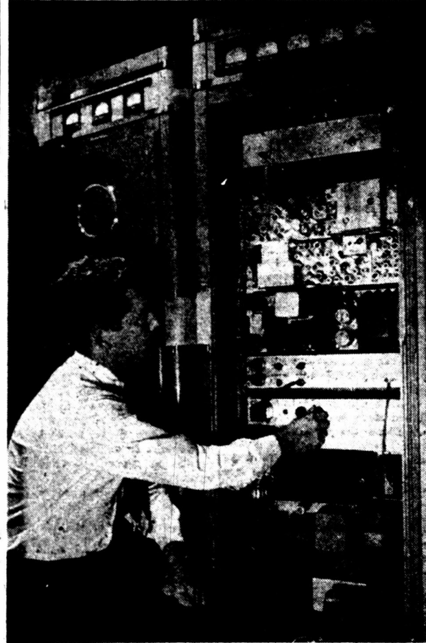
CHECKING THE POWER —Art Joseph, manager of Rotary Engineering Company's electronics department, checks the main transmitting unit in the Big Spring relay station of the concern's new radio telephone communication system. Joseph is turning up a dial to increase the power on the transmitter.
