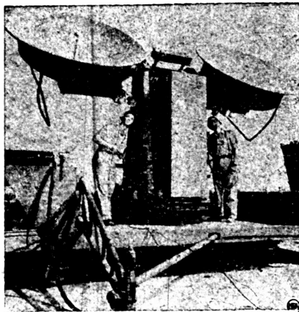
Tracking The Future: The radar unit these men operate at Wallop's Island, Va., provides running record of the 3000-mile-an-hour speed of scale models of planes and rockets.
