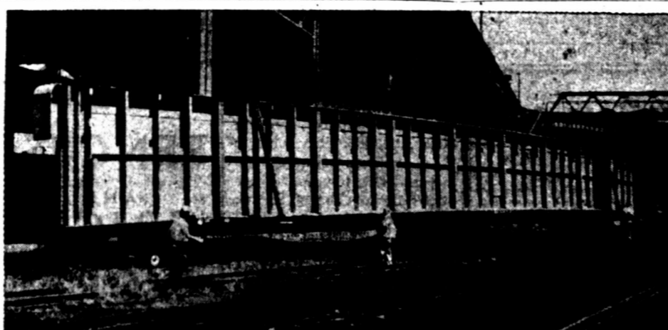
THIS IS REALLY "BIG STEEL"—This giant steel girder, largest single shipment ever to be handled by the New York Central Railway, occupied three flat cars for its trip from New Market, N. J., to New York City. The girder weighs 107 tons, is 153 feet, seven inches long, and 11 feet, five inches high. It is the first of three main girders to be used to build a parkway bridge over New York Central tracks at Woodlawn, in The Bronx.
