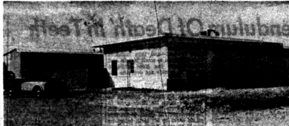
IN NEW HOME —The new home of the Mid-West Lumber Company, at 2010 West Front Street, is pictured above. The dial telephone number is 4-5621. Mid-West handles all builders supplies and materials and will contract to build residential and commercial structures. Joe B. Wright is the manager.
