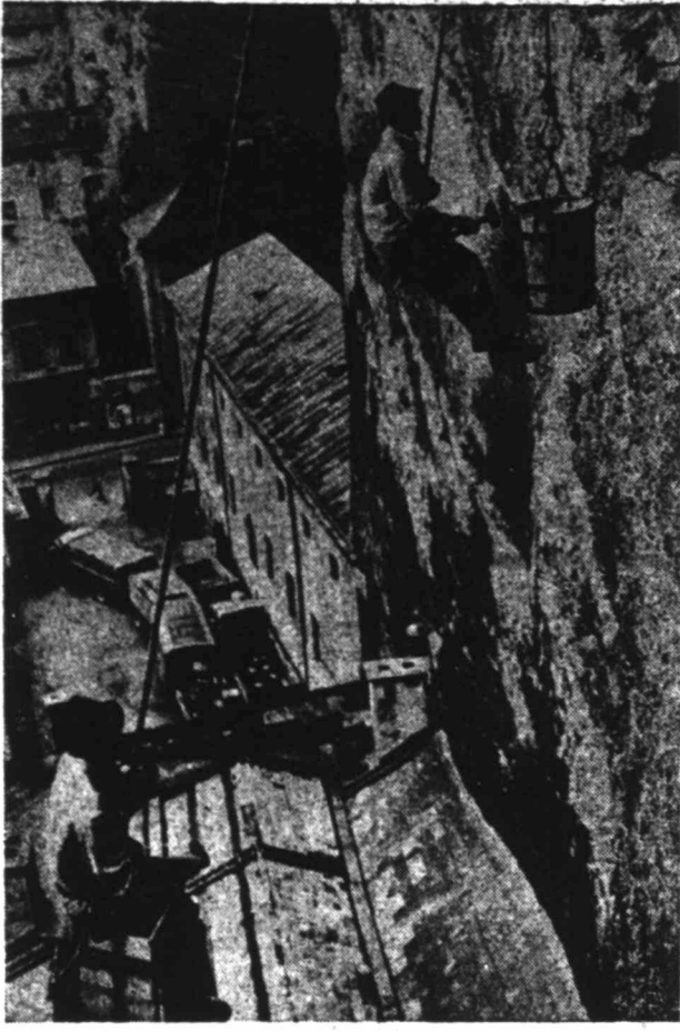
"MOUNTAIN CLEANERS" AT WORK—Working in much the same manner as our city window-cleaners—except with hammers—these "mountain cleaners" at Salzburg, Austria, work over the sides of sheer cliffs above the town. Their job each spring is to check the walls for loosened stones that may endanger life and property below.
