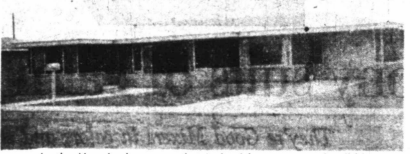
Another idea of a home, recently completed by our construction division.
