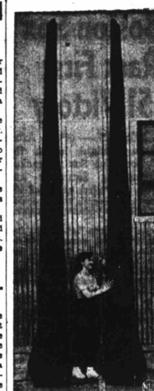
GAS WHAT? — Give up? They're rubber fabric, self-sealing fuel cells that fit into the wings of an Air Force jet fighter. Mary Lee Myers, Firestone Inspector at Akron, O., looks over the long tanks, which immediately seal bullet holes or other punctures.
