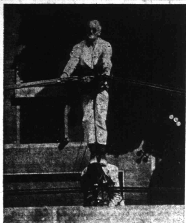
IT KEEPS HIM ON THE JOB —Here's an idea for keeping your workers on the job, boss. Suspended 300 feet above the ground, a steeljacker at the University of California, Berkeley, plants his feet against the shoulders of his partner to help the lower man apply enough force to a drill he's using on the face of a big clock. The steeljacks are repairing a faulty number on the clock's face.
