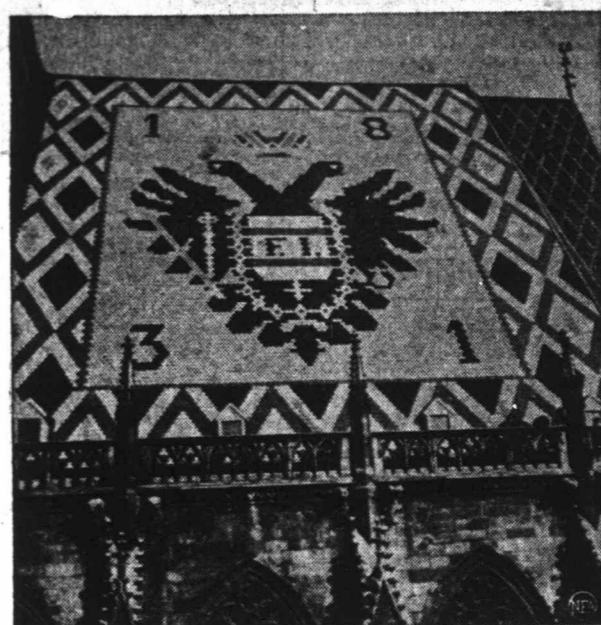
PATTERN FROM THE PAST—The coat of arms of the old Austrian empire is the motif of a novel decorative tile roof just completed on St. Stephen's cathedral in Vienna. The old roof and much of the interior of the 800-year-old church were destroyed during World War II.
