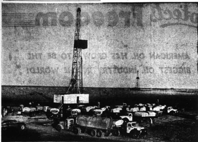
RECORD ACID SHOT IN BENEDUM FIELD-A 40,000-gallon single-stage acid injection was pumped into the Warren Wright and associates No. 1 C. W. Chancellor, Ellenburger producer, in the Benedum field of Central-East Upton County. The Western Company used 17 truck and trailer transports to move the large quantity of chemicals to the location. The chemicals were pumped into the well in two hours and 50 minutes.
