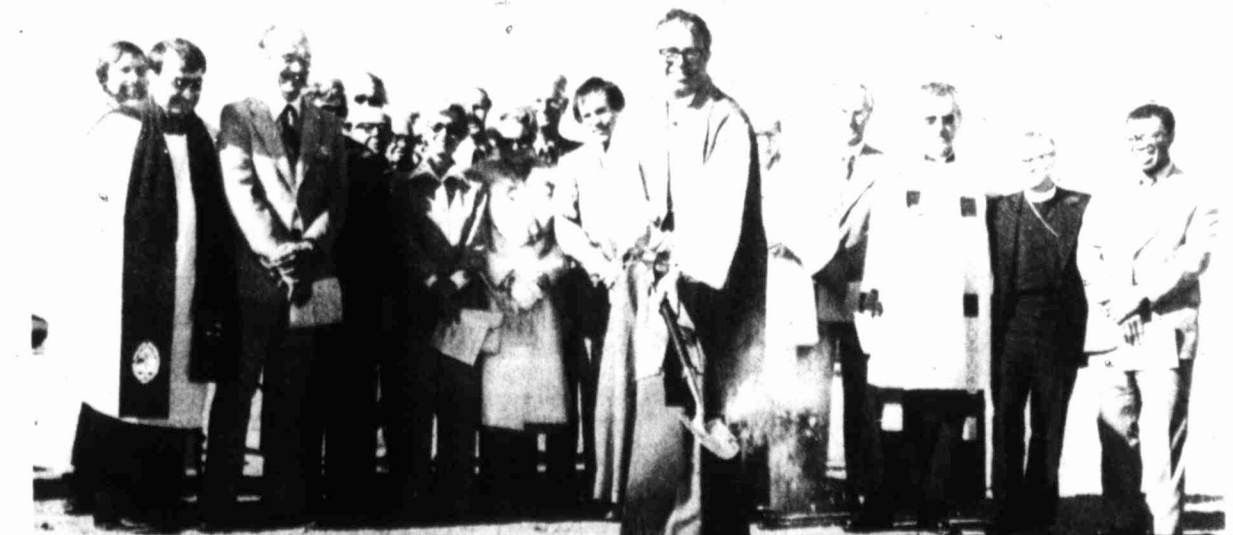
ANOTHER STEP TOWARD COMPLETION — The Rt. Rev. Willis Ryan Henton, Episcopal Bishop from Lubbock, is shown as he breaks the ground for the new retirement center for Big Spring. The center, long a dream of the Rev. Harland Birdwell and parishioners of St. Mary's Episcopal Church, has been named Canterbury, and will be located at 17th and Lancaster. Dignitaries present included the Ven. Richard Wilson, the Rev. Birdwell, the Rev. Jack Monte Jones, and Guilford Jones, who spoke to the crowd about the pre-planning that has gone into the center.
