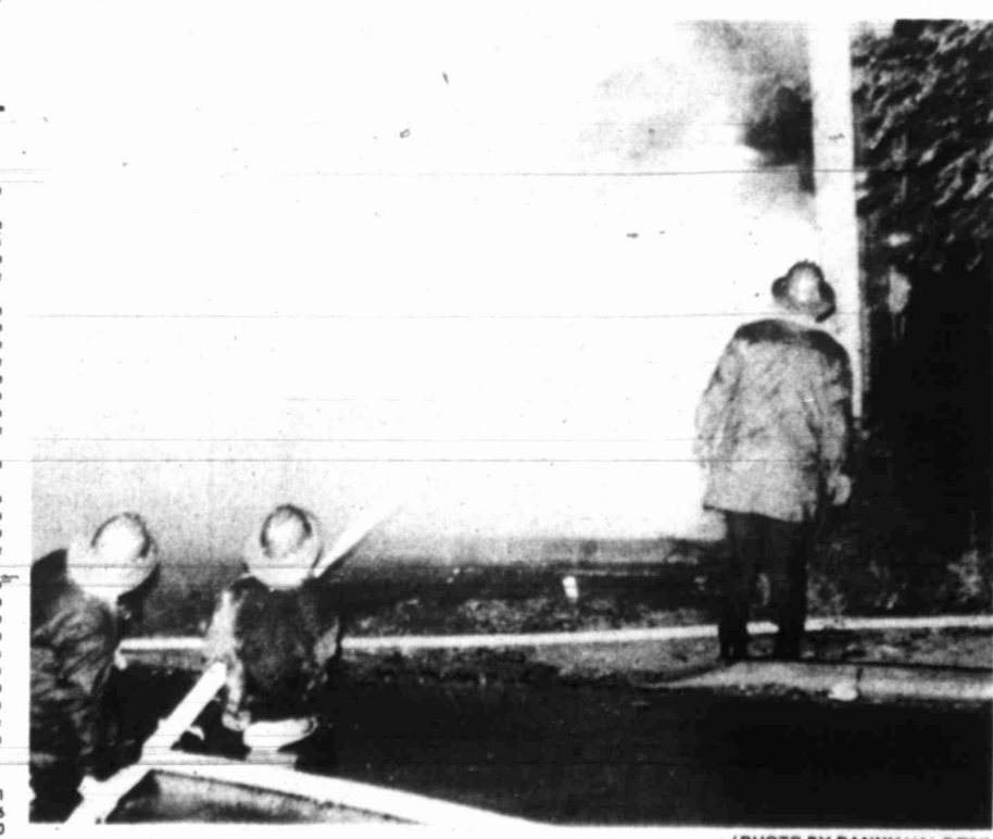
LOUNGE BURNS — Approximately 30 firemen and five fire trucks fought flames at what used to be the Blue Moon Lounge early this morning after arsonists started the fire in a vacant part of the building.
