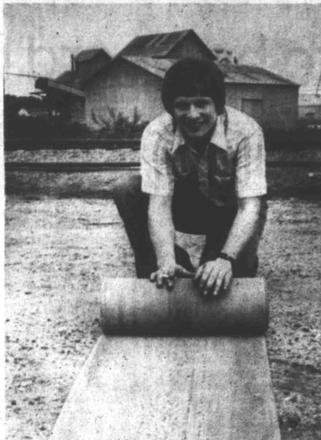
CHIP AT WORK — President Carter's son Chip, 27, rolls the conveyor belt, that he helped warehouse workers haul from the roof of the three-story Carter peanut warehouse. Wednesday was Chip's first day working at the Plain's warehouse.
