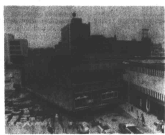
(AP WIREPHOTO) NO SMALL MOVE FOR OLD STORE — Liebermann's Jewelry Store, up off its old foundation, left, and sitting ominously in middle of street in Joliet, Ill., is moved ever-so-slowly from one corner to another. The job to move the 800-ton building will cost the owner $100,000, and take more than a month to complete. However, a new structure would cost $450,000. Back of building is to be swung around to site parallel to building at right.
