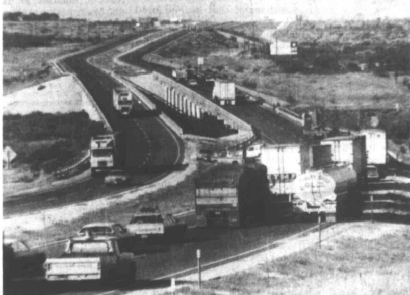
BRIDGE BLOCKED — An accident occurred on this bridge on IS 20 west of Big Spring this morning between a truck and a farm tractor which halted traffic on the highway for over an hour before one lane of the bridge could be cleared.
