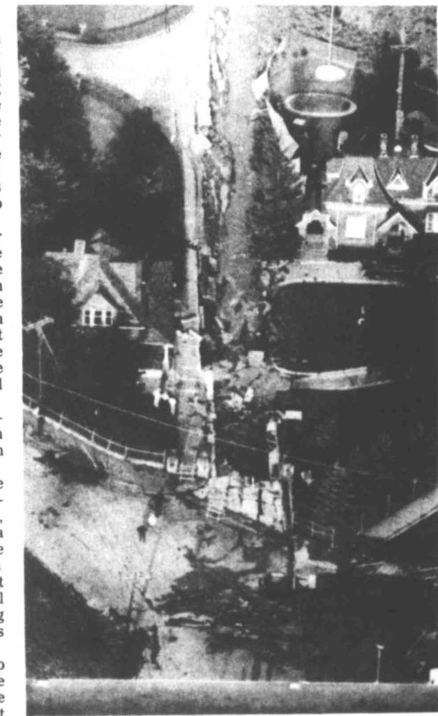
(AP WIREPHOTO) SEWER EXPLOSION — One street was destroyed and several damaged early Thursday morning as a sewer line exploded and rocked a wide area of Akron's west side. Damages will be in the millions of dollars, some residents were evacuated and there were no injuries.
