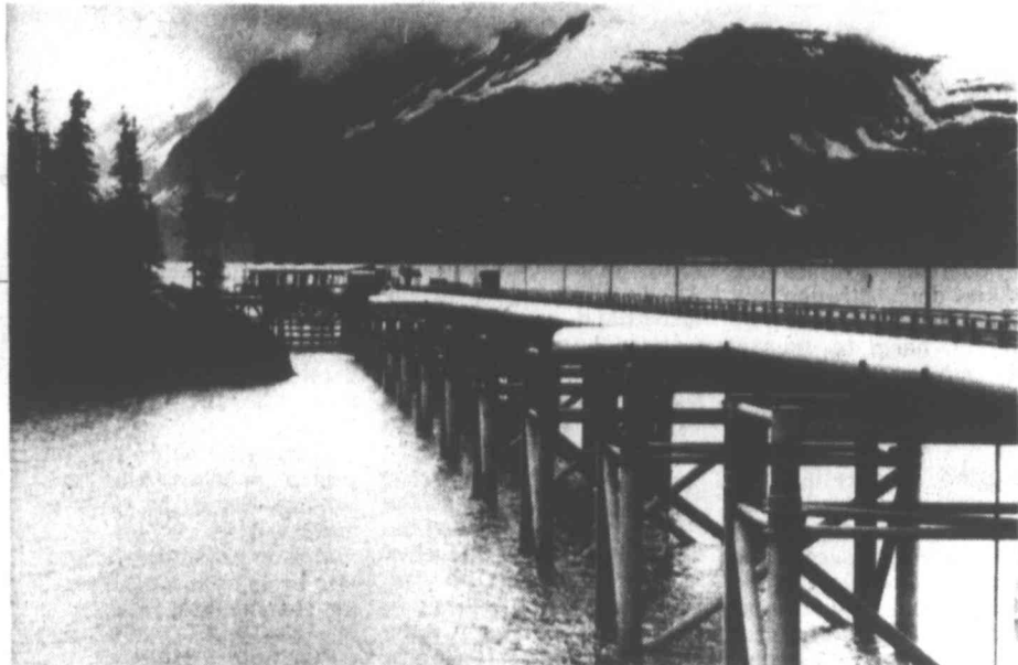
PIPELINE TANKER BERTH — This is one of four tanker berths built to accommodate supertankers carrying trans-Alaska pipeline oil. The pipe on the berth leads to storage tanks built along the shoreline. The city of Valdez is several miles away across the bay.
