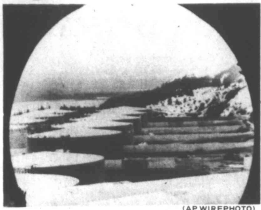
PIPE'S EYE VIEW — This view, taken from inside a piece of pipe, shows oil storage tanks at the terminal near Valdes, of the trans-Alaska pipeline. The storage tanks can hold up to six days of oil in case the pipeline has to be shut down for any reason.
