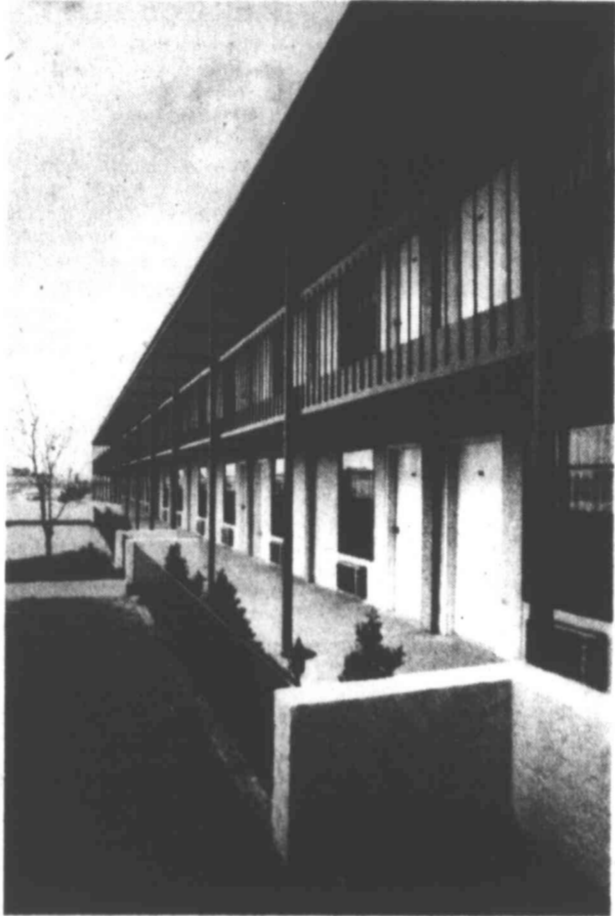
VIEW FROM THE COURTYARD Complex on city's north perimeter
