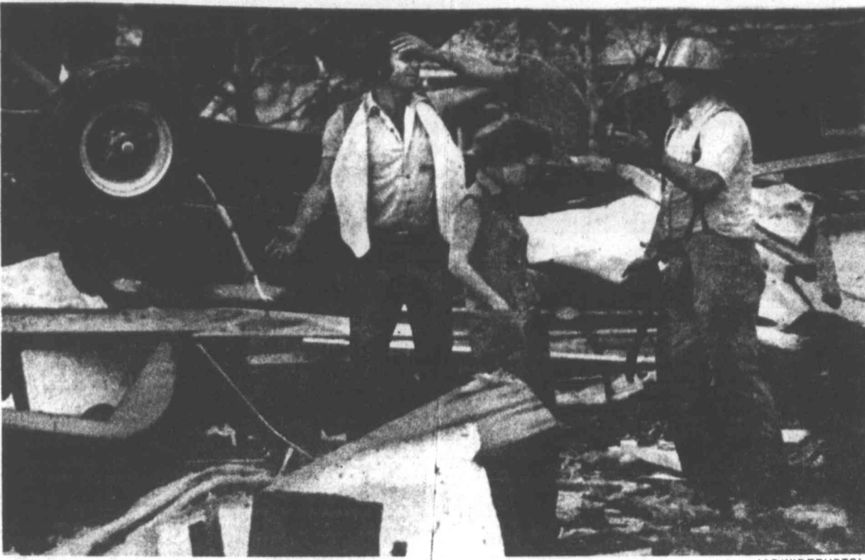
TORNADO DAMAGE — A Pleasant Hill couple talk with a rescue worker as they stand in the wreckage of their mobile home after a tornado swept through the
