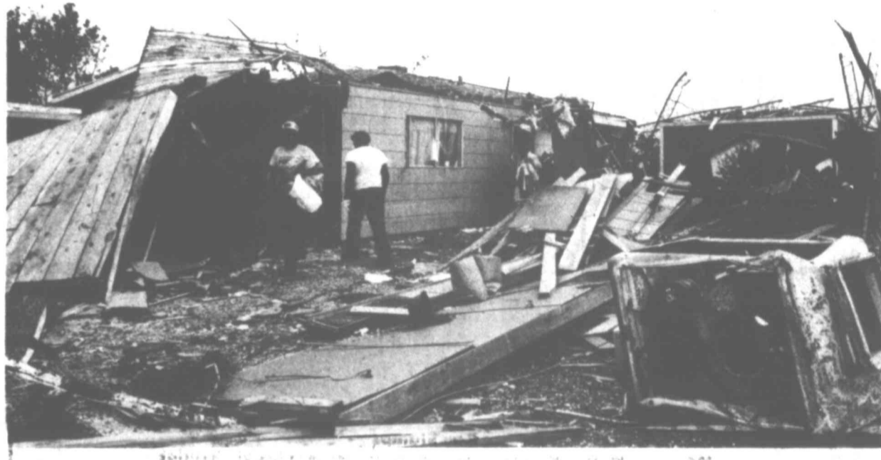
HEAVY DAMAGE — The winds trashed homes lining 3rd St. just north of the hospital, tearing roofs away and hurling debris through doors and windows.
