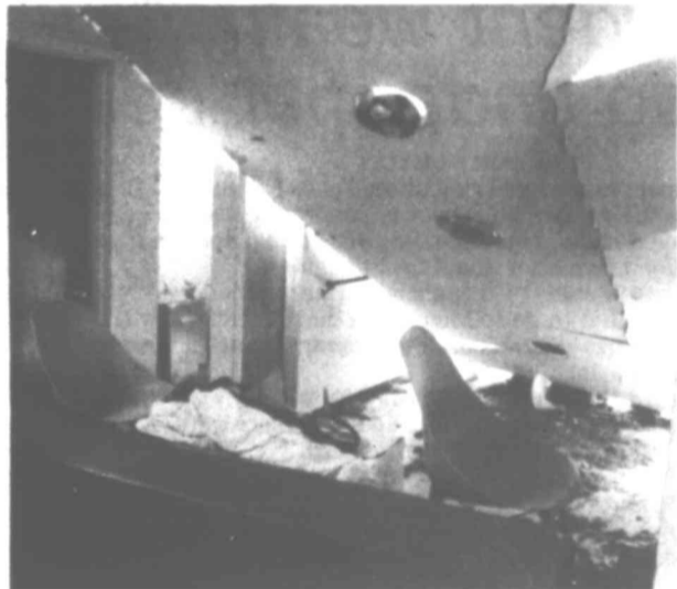
NURSING HOME — The Monahans Convalescent Home housed almost 50 people, according to administrator Julie Martinez. Five minutes before the tornado hit, she herded the residents into the halls, where they waited huddled together for the storm to pass. The residents were later sent either to relatives in Monahans or to other homes in Kermit.
