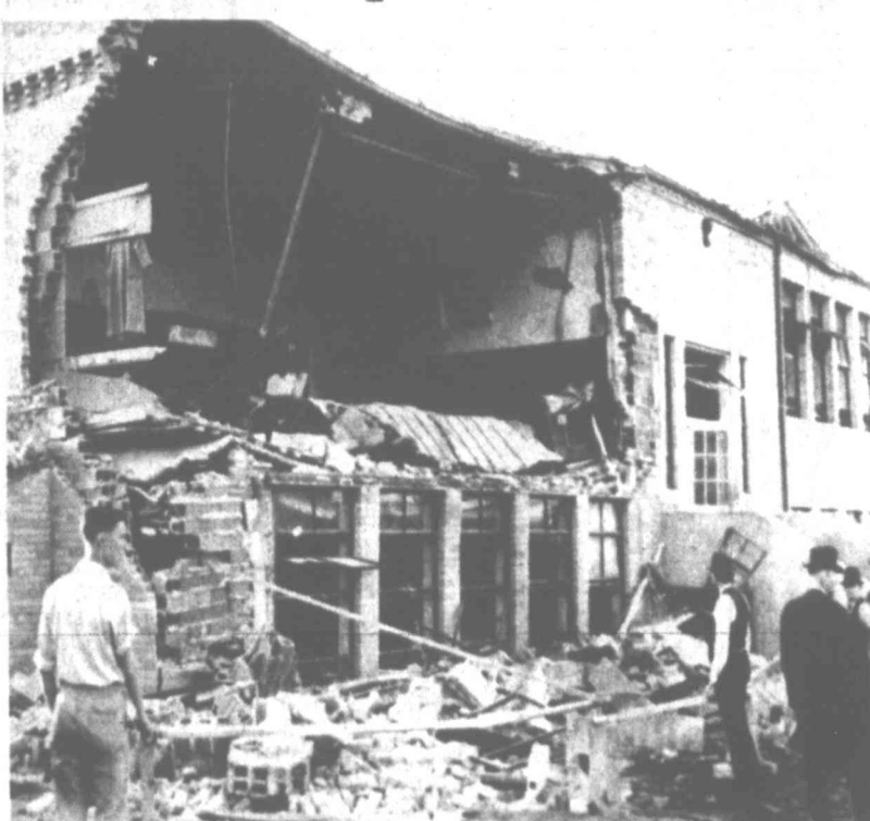
SCHOOL BLAST — It was 40 years ago today — March 18, 1937, that a blast caused by leaking natural gas ripped through a school building at New London, Tex., killing almost 300 students. Here workers comb through the wreckage of the building searching for victims.
